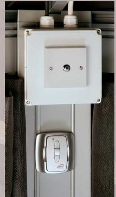
Lighting Control Box with integral Dimmer Switch
